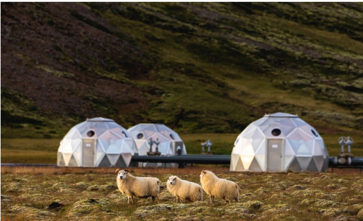
Figure 1: To achieve permanent mineralization of carbon dioxide – turning carbon dioxide into stone – Carbfix uses three injection wells near the Hellisheiði geothermal power plant in Iceland to inject carbonated water into underground rock formations, where it mineralises in less than two years. The stored carbon dioxide is captured from two sources: the emissions of the geothermal power plant, and the atmosphere through direct air capture. Photo from Carbfix.
